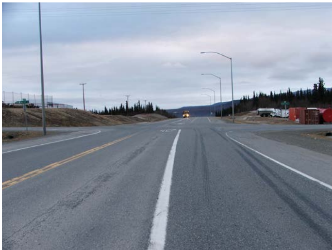
Intersection of Healy Spur Road and George Parks Highway-Northbound
