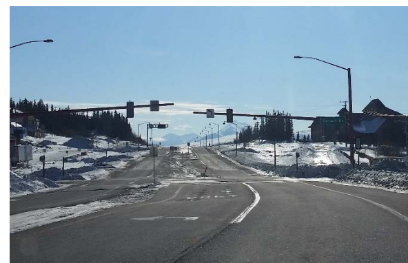
Nenana Canyon intersection, Parks Highway
